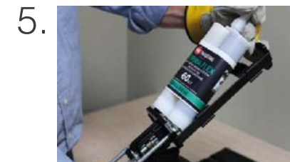
5. Place the cartridge in the spray gun
