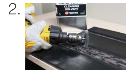
2. Roughen the working surface
