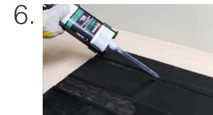
6. Apply Permaflex repair material
