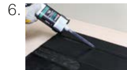
6. Apply Permaflex repair material
