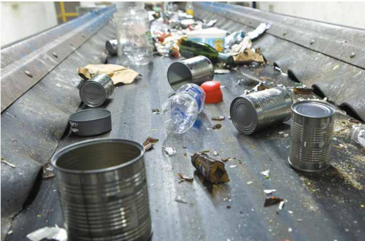
oil resistant conveyor belts in use in a recycling plant
