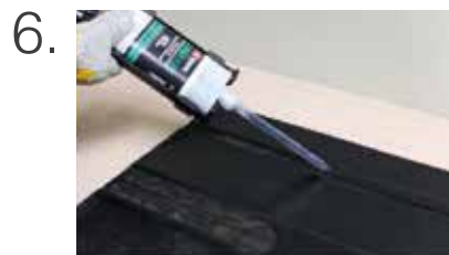
Apply Permaflex repair material
